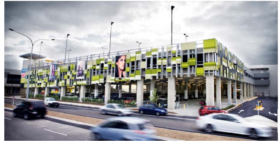
New three-level carpark viewed from Ferguson Street
