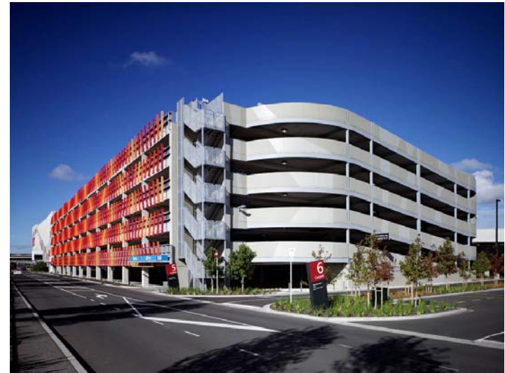
North-east multi-storey carpark
