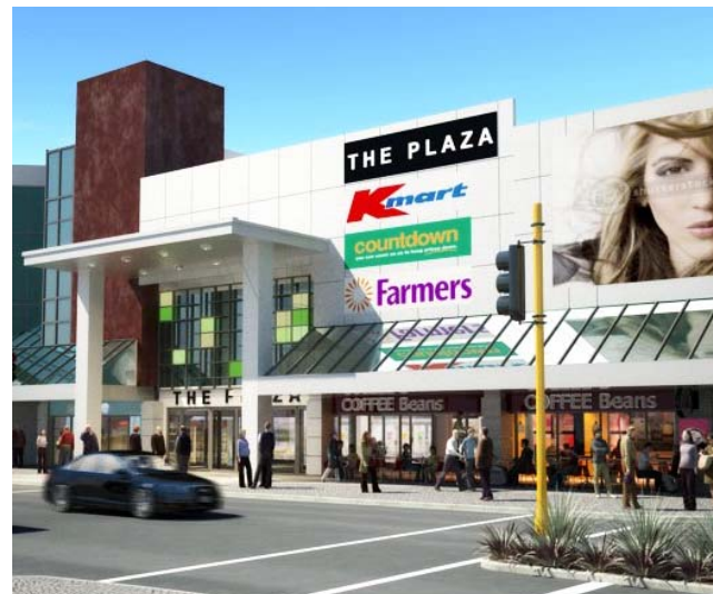
Artist impression of Church St entry The Plaza Shopping Centre, Palmerston North
