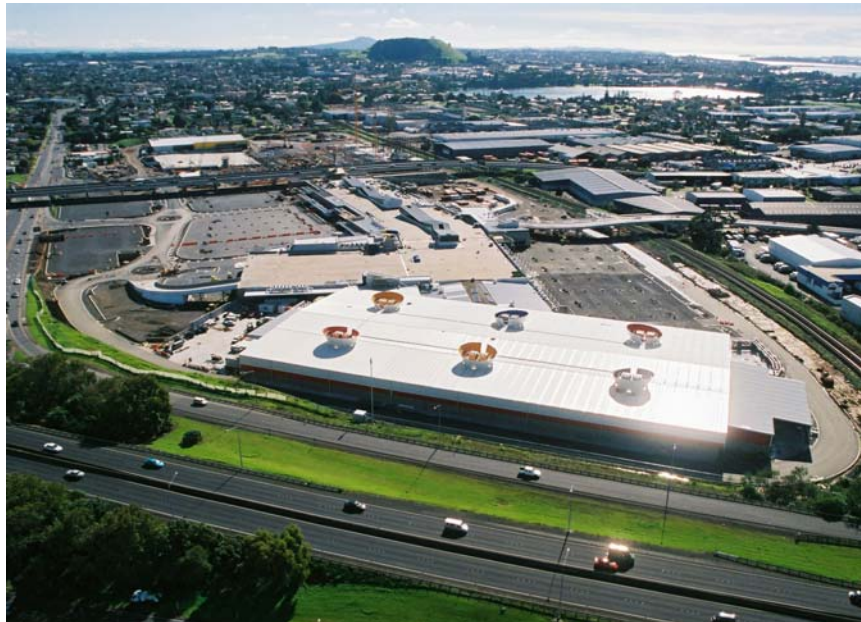
View North – Stage I & II
